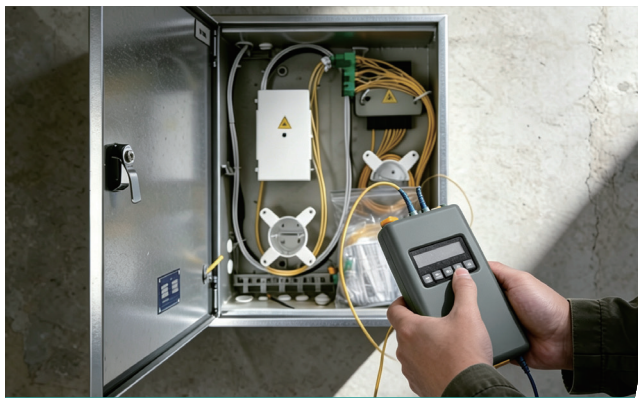
PRIMARY SPLITTER VERIFICATION
